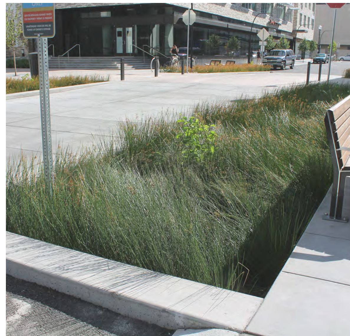
Natural drainage channel
