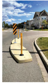
Photo of an adaptable curb extension on Allard Boulevard & Anthony Crescent, as part of the Allard Street Lab.
