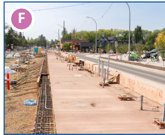
Area 3: Glenora Stop concrete work
