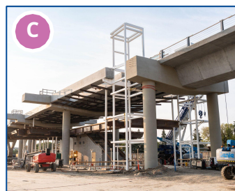
Area 6: WEM Station construction
