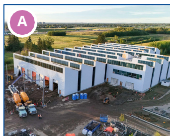
Area 8: Lewis Farms Storage Facility construction
