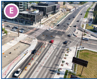
Area 4: SPR/142 St intersection open
