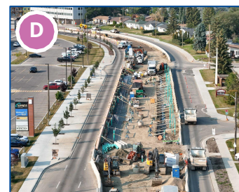
Area 5: Meadowlark Stop underground drainage
