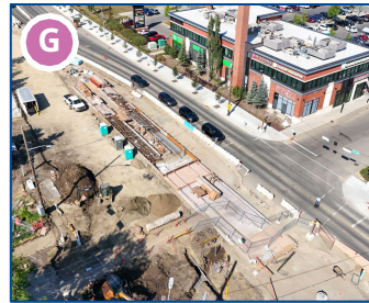
Area 2: 104 Ave track & road work
