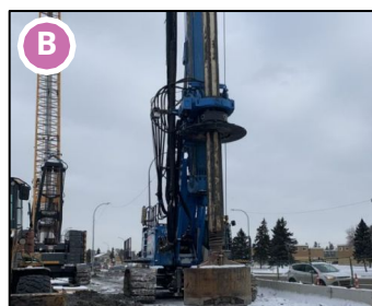
Area 6 - Elevated Guideway piling on 170 Street
