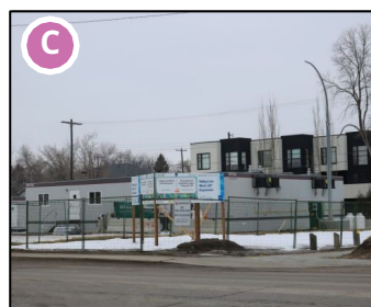
Area 4 - Site Office / Laydown Yard on 143 Street and Stony Plain Rd.
