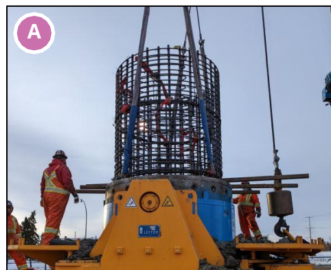
Area 6 - Elevated Guideway piling on 87 Avenue
