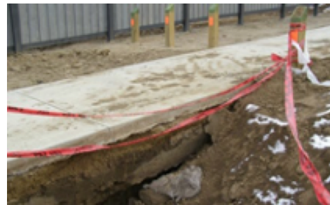
Undermined sidewalk
