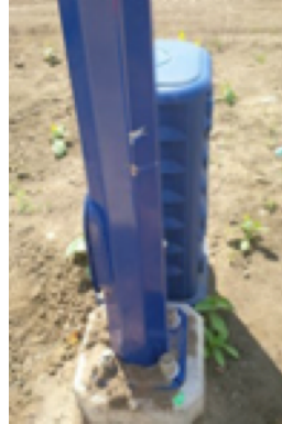
Galvanizing damage
