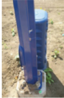
Galvanizing damage
