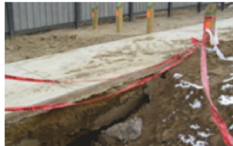
Undermined sidewalk
