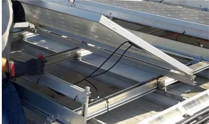
Figure 9 - Module Connectors
