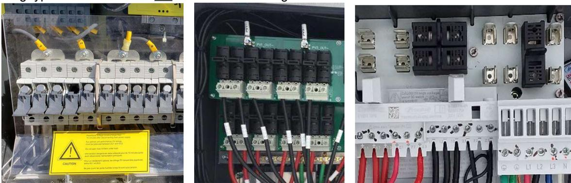
Figure 15 – Examples of DC String Fuse Holders
