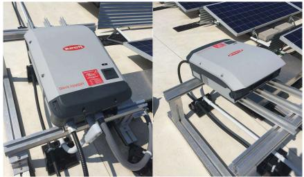
Figure 12 – Example Inverter Mounting Structure (prior to shade cover installation)
