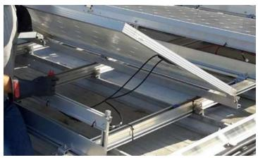
Figure 9 - Module Connectors
