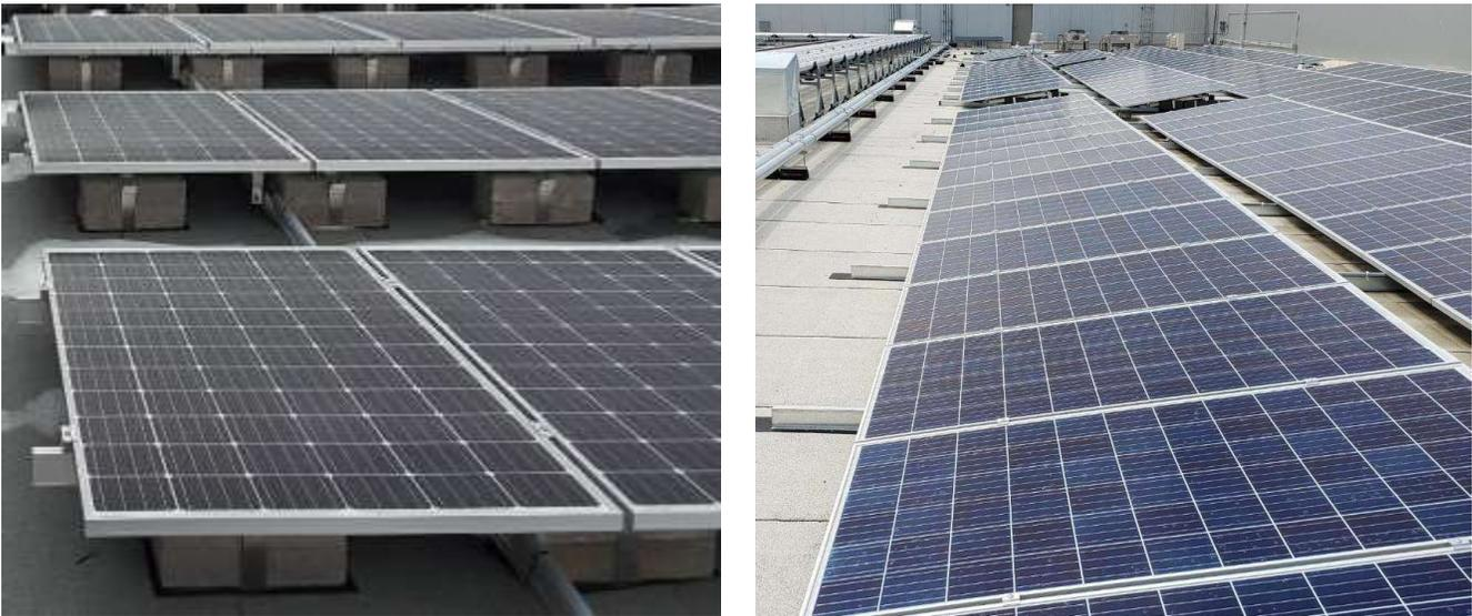
Figure 7 - Ballasted Racking Solution
