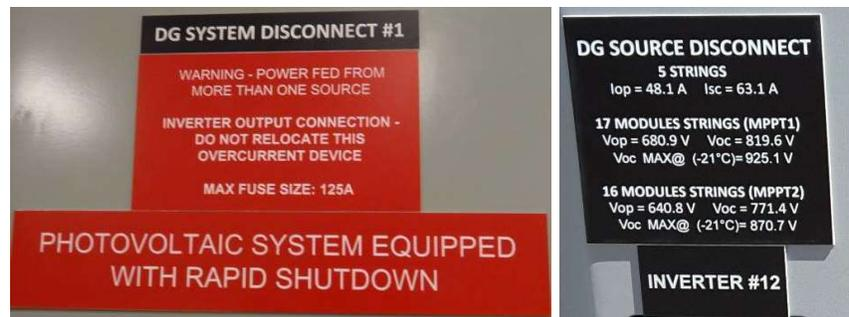
Figure 18 - Equipment Labeling (Sample)
