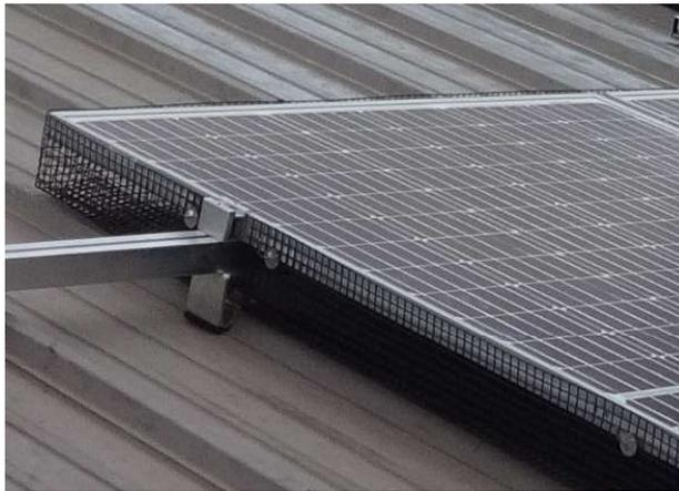
**Figure 15 – Wire Mesh for Rodent Protection**
