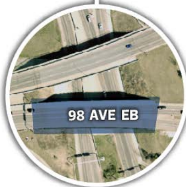
98 Avenue Bridge eastbound over Connors Road
