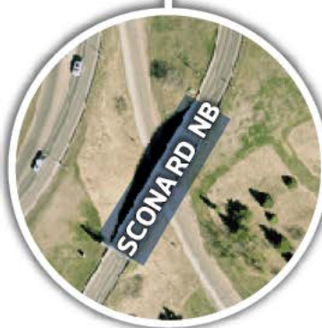
Scona Road Bridge northbound over Connors Road
