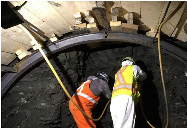
Figure 2a: NEST NC2/NC3, Undercut Excavation
