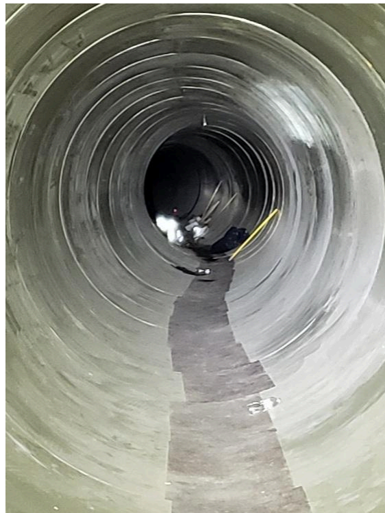
Figure 2b: SESS SW4 Completed Tunnel with Liner
