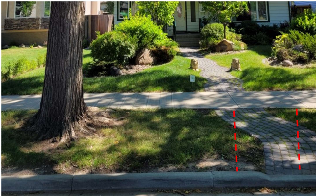
Figure 3. Approximate Location of Open Excavation.
