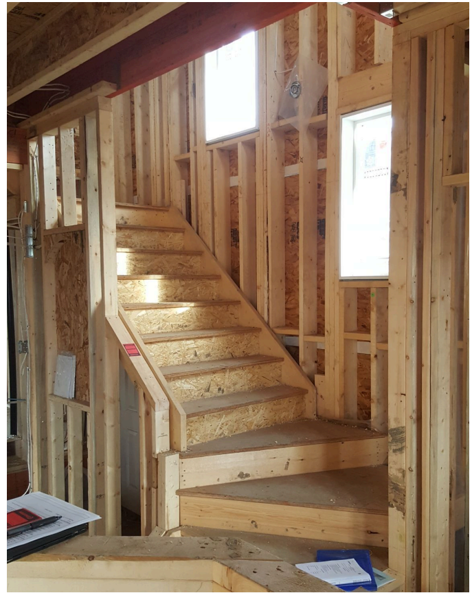
No guard, no 3 point contact
