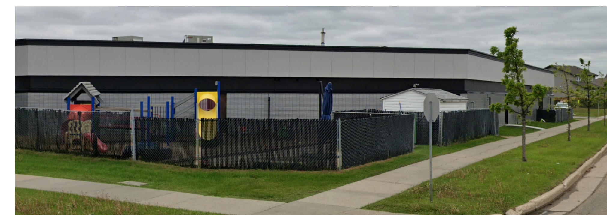
Photograph of existing conditions from intersection of 127 Avenue and Hermitage Road
