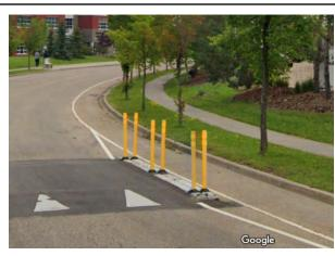
The example shown is of a permanent asphalt speed table. The Street Lab will use rubber speed humps.
