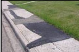
Asphalt patching
