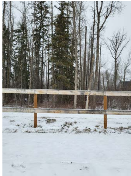
Post and Rail fencing require wood stain
