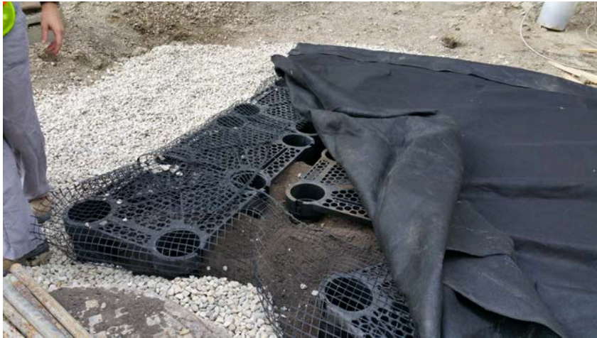
Soil Cell Installation
