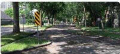
Chicanes are a series of offset curb extensions in the road that are added to reduce speed.
