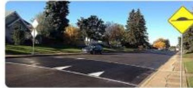
Speed humps are a raised section of the road. They are similar to raised crosswalks but are shorter in length and not placed at crossings.
