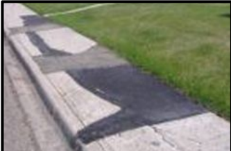
Asphalt patching
