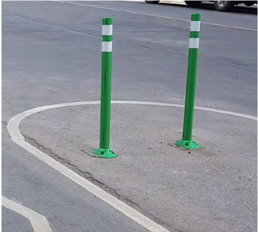
36A Avenue - Example image of flexible bollards
