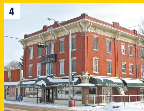
4 6423 – 112 Avenue (1913) Gibbard Block The historic Gibbard Block, home to La Bohème Restaurant, is a prominent architectural feature of the Highlands business district.
