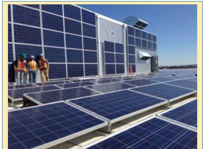
Environment Canada's Eastgate office building in Edmonton is covered by a 153.75 kW solar panel array that was installed in 2013.
