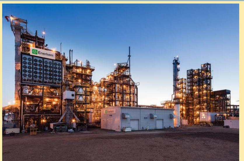
The **Enerkem Alberta Biofuels facility** plant is a full-scale biofuel production facility taking municipal solid waste from Edmonton and producing ethanol and methanol. This facility is the first to ever sell its ethanol under the United States Renewable Fuel Standard. Over 100,000 metric tonnes of solid waste are diverted from Edmonton landfills every year.
