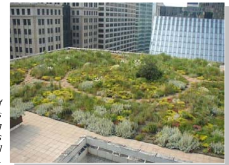
The green rooftop of Chicago City Hall moderates extremes in building temperature and reduces stormwater runoff, as well as providing amenity space.
