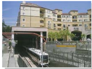
Holly St. Transit Oriented Village in Pasadena, California.
