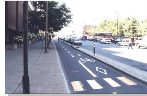
Sidewalk, bike lane and roadway share the same street.
