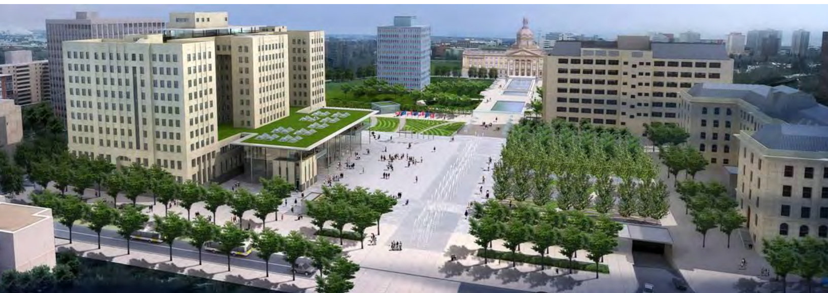
Image courtesy Carlyle + Associates
