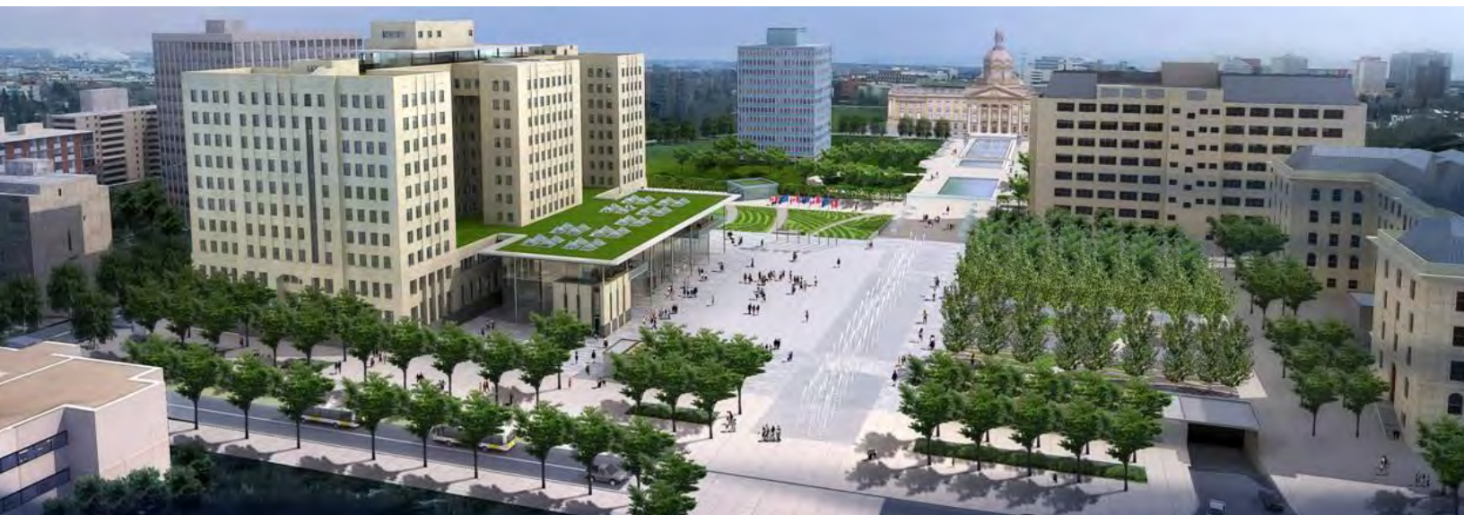
Image courtesy Carlyle + Associates
