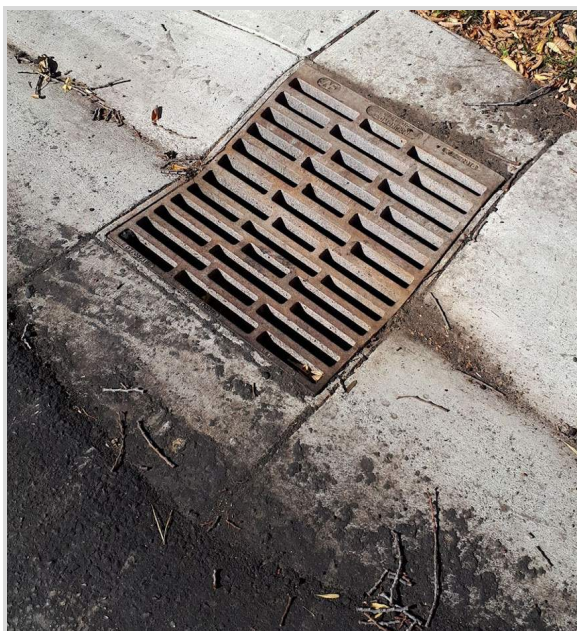
Figure 3.27A - Example of bicycle-friendly catch basin design
