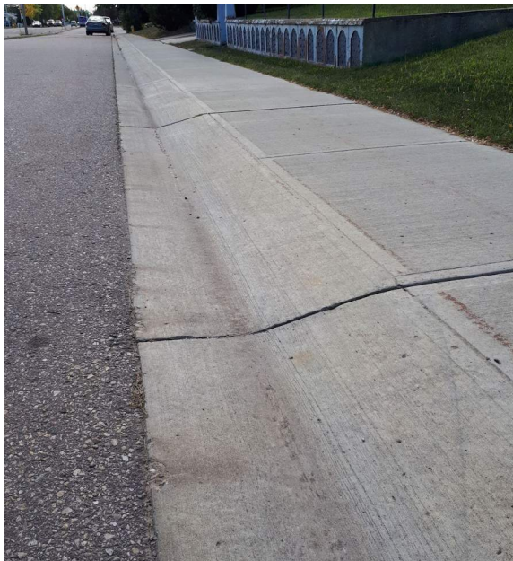
Figure 3.25 Rolled Face Curb
