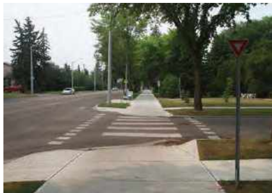
Figure 3.75: Crossride Treatment for use with Shared-Use Path
