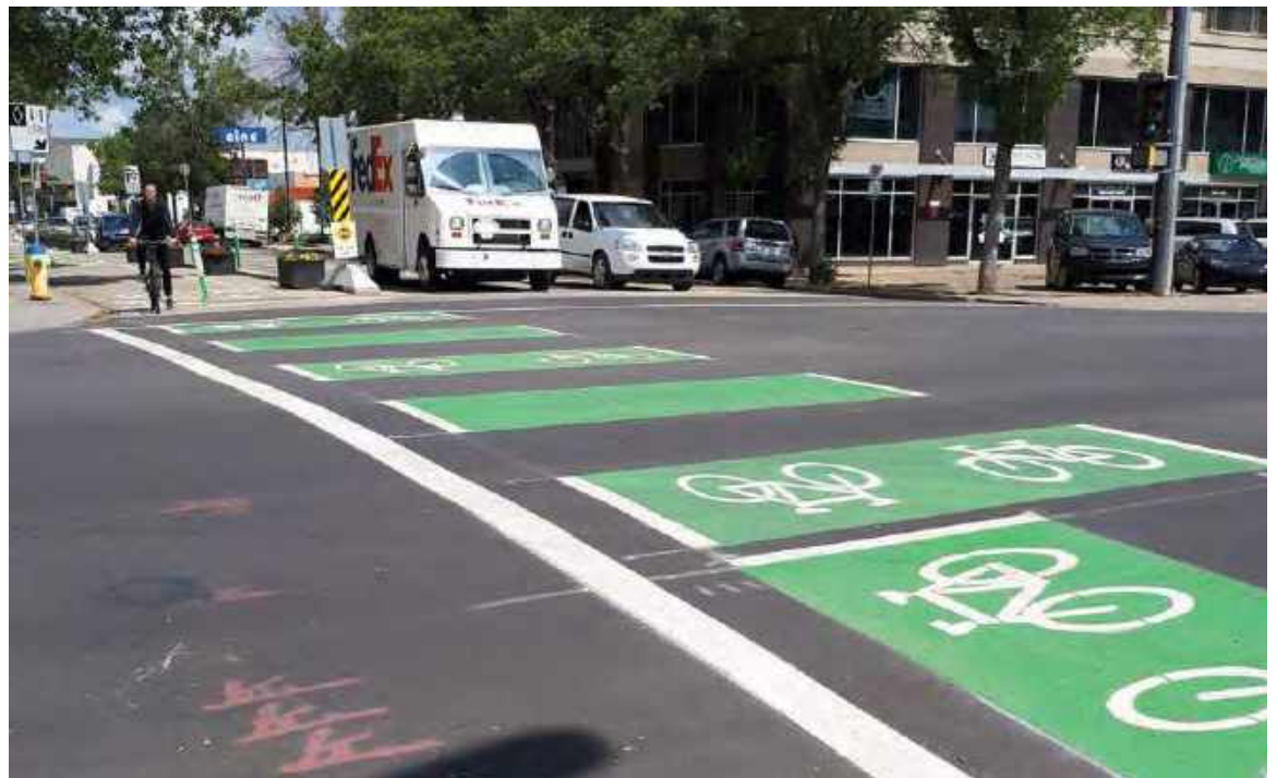
Figure 3.76: Green Coloured Conflict Marking Pavement Treatment
