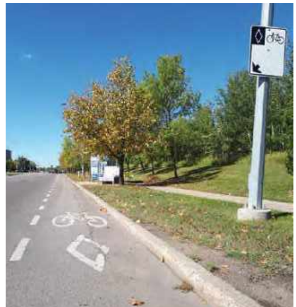
Figure 3.22 Painted Bike Lane at Curbside Transit Stop
