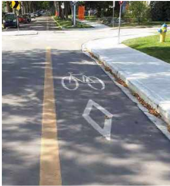
Figure 3.24 Contraflow Bicycle Lane Line
