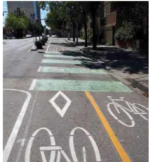
Figure 3.24 Contraflow Bicycle Lane Line
