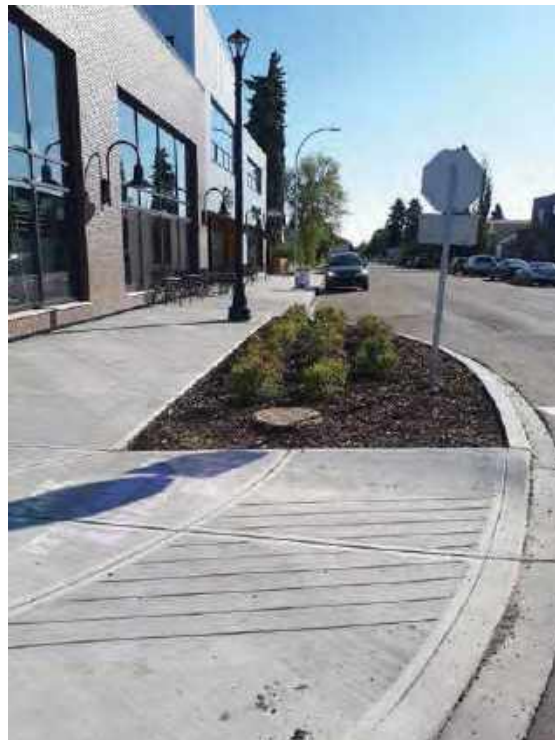
Figure 3.32 Curb Extension in Ancillary Zone
