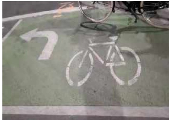
Figure 3.77 Two-Stage Turn Queue Boxes
