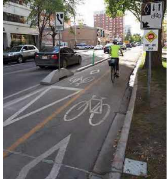
Figure 3.13 Bidirectional Protected Bike Lane
