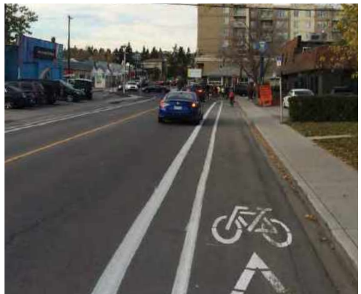
Figure 3.16 Painted Buffered Bike Lane (Source: City of Calgary)
