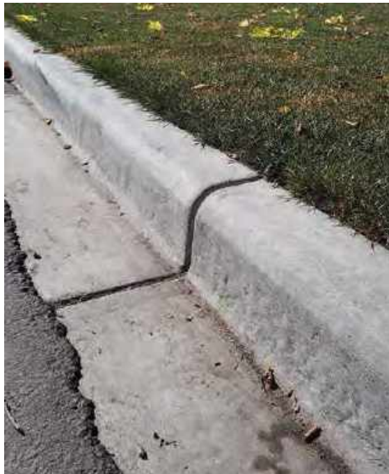
Figure 3.26 Straight Face Curb
