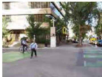
Figure 3.58 Two-Stage Left Turn Queue Boxes
