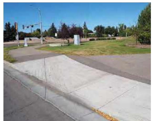
Figure 3.62: Bike Ramp from On-Street Bike Lane to Off-Street Bike Path or Shared-Use Path
