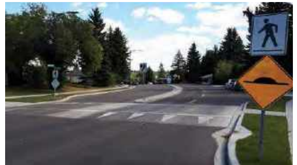
Figure 3.81 Raised Crosswalk
