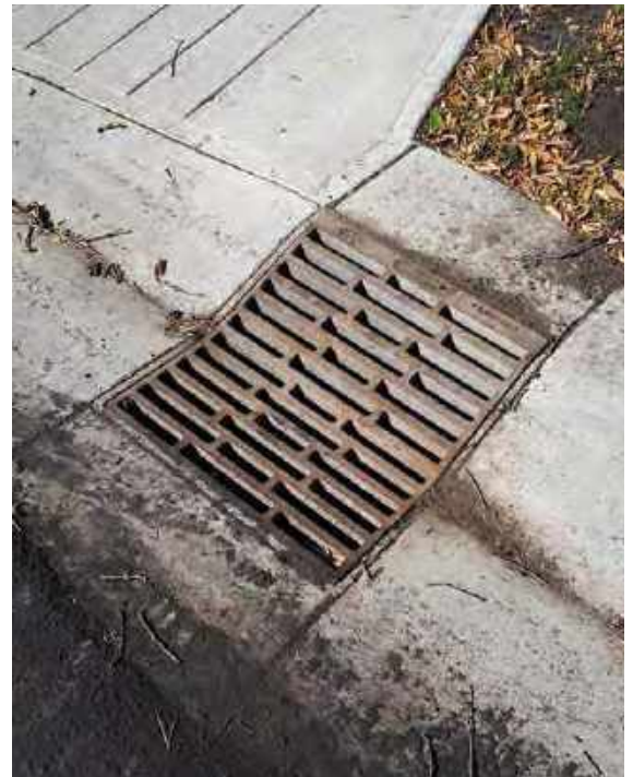
Figure 3.29 - Example of bicycle-friendly catch basin design
