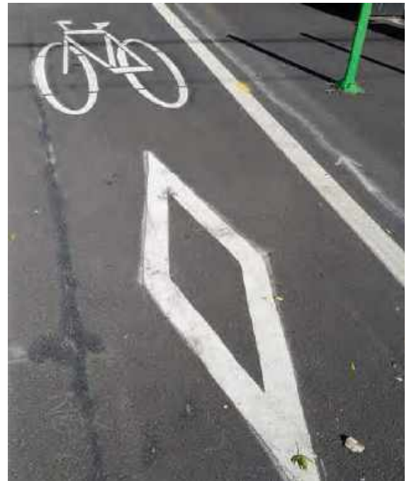
Figure 3.23 Reserved Lane Pavement Markings for Bicycle Lanes
