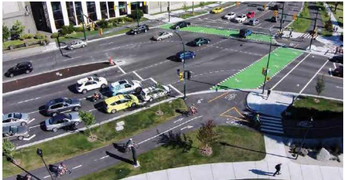
Figure 3.59: Protected Intersection (Source: City of Vancouver)
