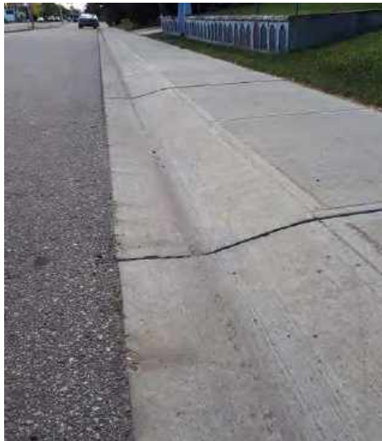
Figure 3.28 Roll Face Curb
