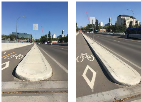
Figure 3.14 Protected Bike Lane Delineators
