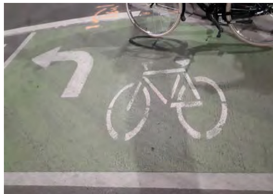
Figure 3.77 Two-Stage Turn Queue Boxes
