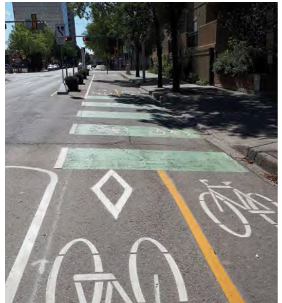
Figure 3.24 Contraflow Bicycle Lane Line
