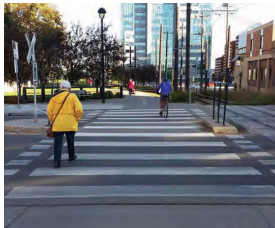
Figure 3.65: Mid-Block Shared-Use Path Crossing
