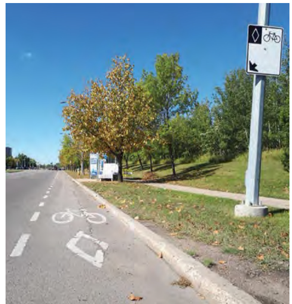
Figure 3.22 Painted Bike Lane at Curbside Transit Stop
