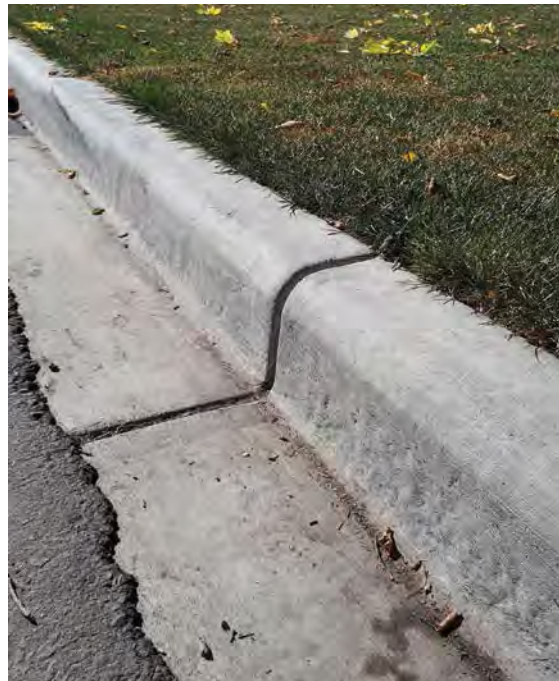
Figure 3.26 Straight Face Curb
