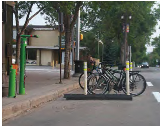
Figure 3.35 Bicycle Parking Corral in Ancillary Zone
