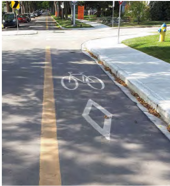
Figure 3.24 Contraflow Bicycle Lane Line
