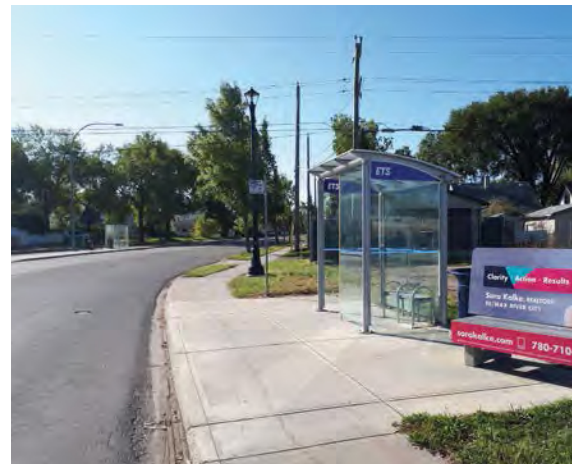
Figure 3.36 Transit Shelter (with sidewalk access and shelter oriented to protect waiting passengers from prevailing winds)
