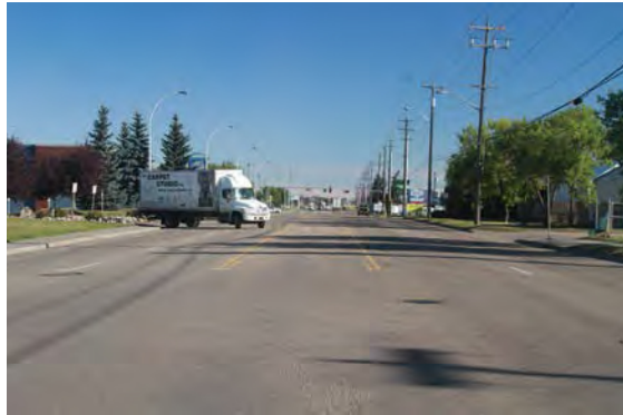
Two-way or shared left-turn centre lane (Typically only used in industrial area arterial streets)
