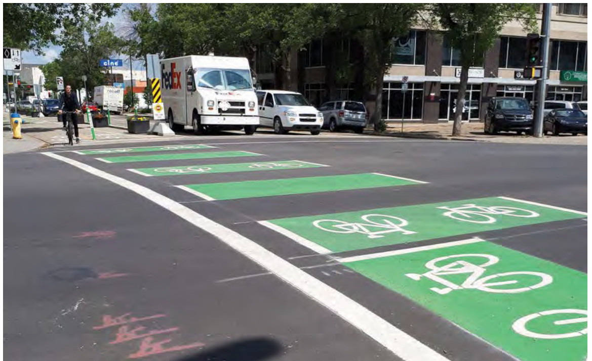
Figure 3.76: Green Coloured Conflict Marking Pavement Treatment
