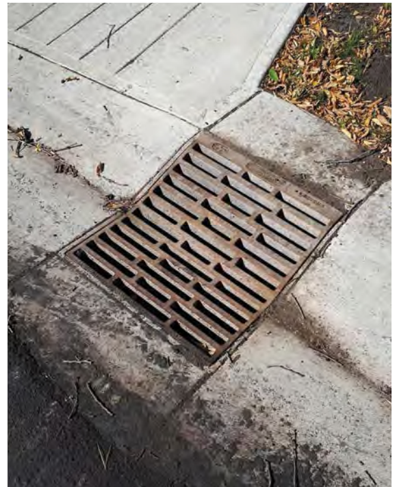
Figure 3.29 - Example of bicycle-friendly catch basin design
