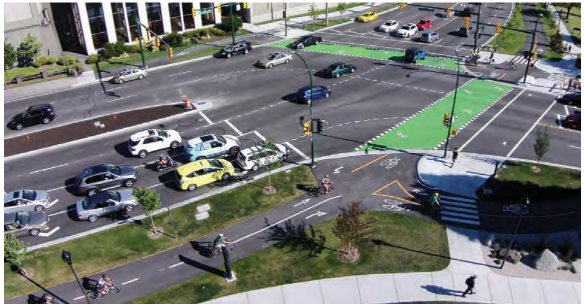
Figure 3.59: Protected Intersection (Source: City of Vancouver)
