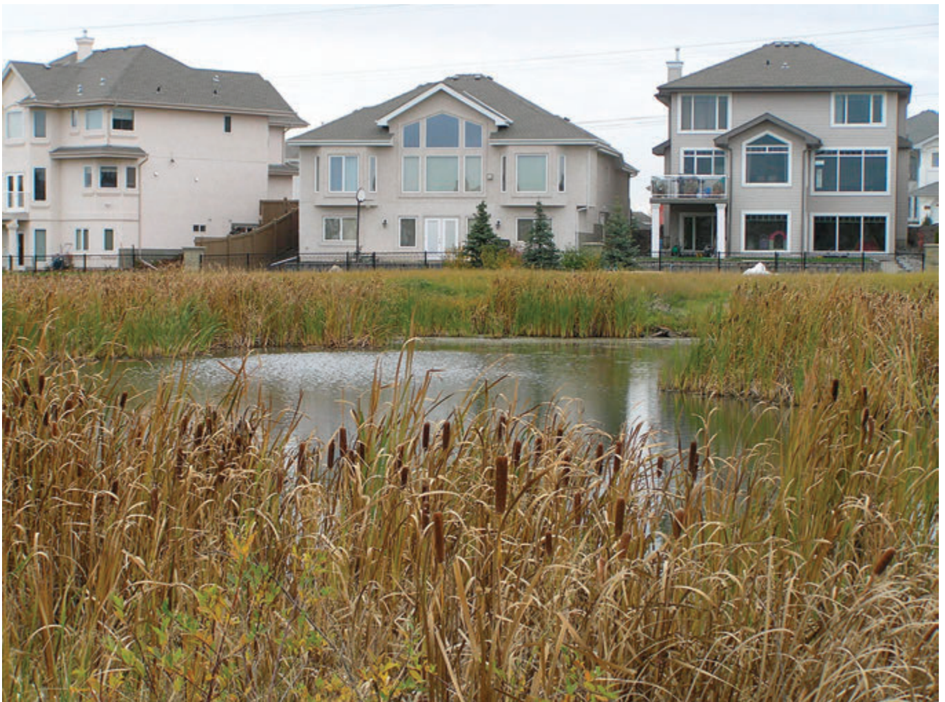
LOW IMPACT DEVELOPMENT USES CONSTRUCTED WETLANDS IN NEW COMMUNITIES AS ONE STRATEGY TO CAPTURE AND TREAT RUN-OFF.
