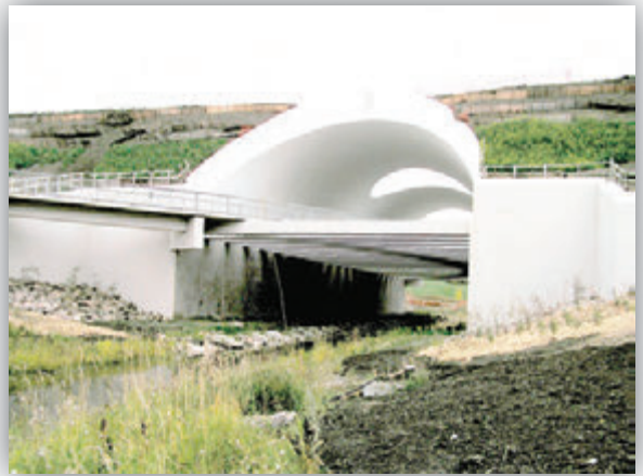
THE ANTHONY HENDAY WILDLIFE PASSAGE FEATURES A VEGETATED BRIDGE UNDERPASS, NATURAL LIGHTING, AND AN INTEGRATED PEDESTRIAN PATHWAY.
