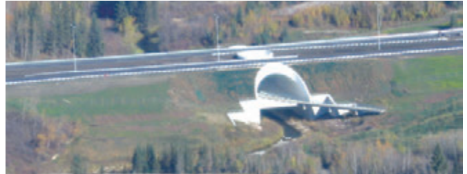
ANATURALIZEDCORRIDORUNDERAMAJORHIGHWAYPROVIDESAPASSAGE FORWILDLIFEANDMAINTAINSECOLOGICALCONNECTIVITY.ITFEATURES A VEGETATED UNDERPASS, NATURAL LIGHTING, AND AN INTEGRATED PEDESTRIAN PATHWAY.
