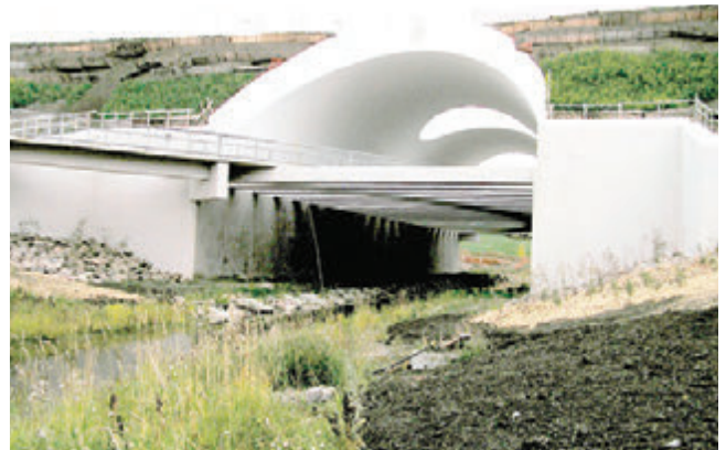
ANATURALIZEDCORRIDORUNDERAMAJORHIGHWAYPROVIDESAPASSAGE FORWILDLIFEANDMAINTAINSECOLOGICALCONNECTIVITY.ITFEATURES A VEGETATED UNDERPASS, NATURAL LIGHTING, AND AN INTEGRATED PEDESTRIAN PATHWAY.
