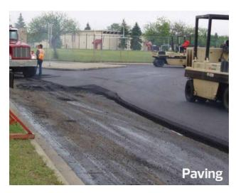
Paving is the quickest step. Contractors can usually pave 3–5 blocks per day.
