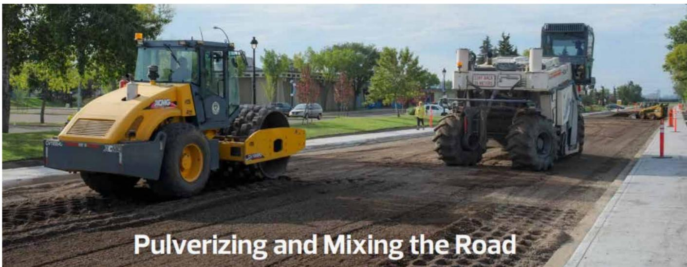
The graded road base needs two to three days for it to cure prior to paving and can be driven on. The road will be fully closed during paving operations and typically opens later on the same day.
