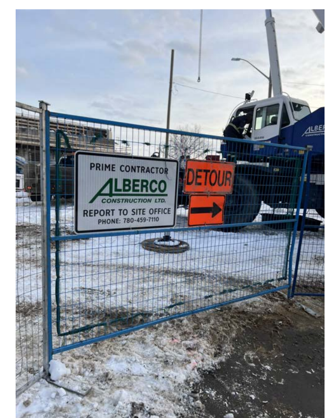
Alberco Site Signage, "Detour" w/ Arrow Sign On each side of 82 Ave for the "U" shaped diversion of pedestrian walkway. Walkway width min. 1.5m.
