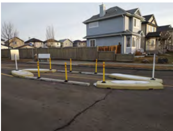
Adaptable Centre Median
