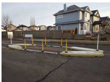
Example of an adaptable centre median
