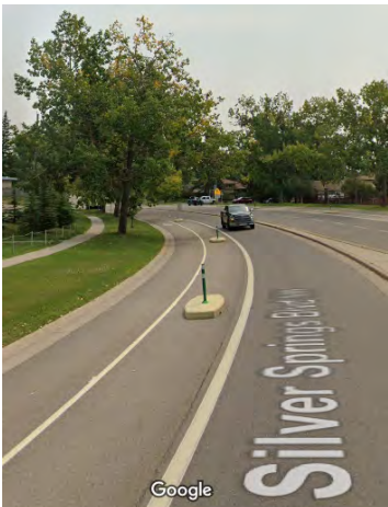
Above is a photo of a one-way protected bike lane where there is no parking - located on Silver Springs Boulevard in Calgary, AB
