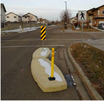
Example of an adaptable curb extension
