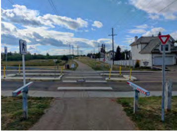
Example of an adaptable two-stage crossing
