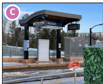
Area 3 - Muttart Signage and Security Camera Installations
